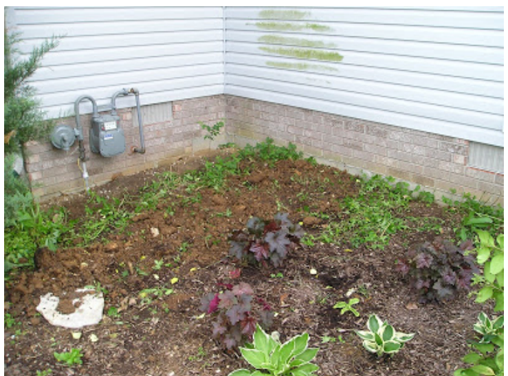
After the shrub is removed, the meter is now accessible
