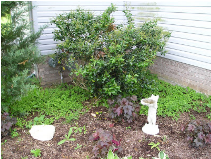
The gas meter is hidden behind this shrub
